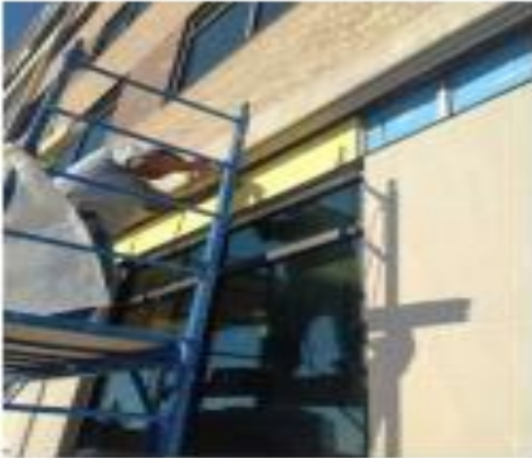
Dens Glass being applied over Hat Channel
