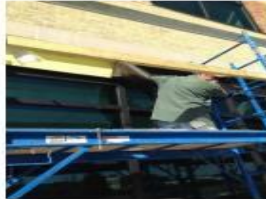
Vapor Barrier being installed over Dens Glass
